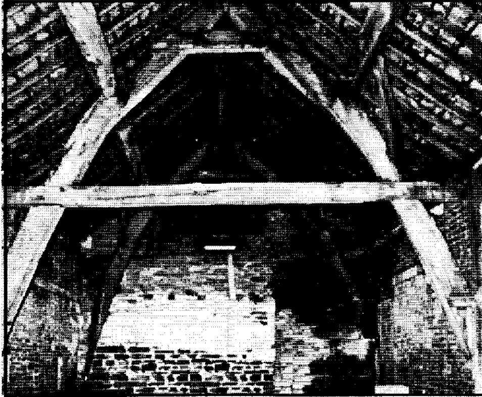
Photo showing the giant oaken "crucks" made from the natural curve of England's precious timber
