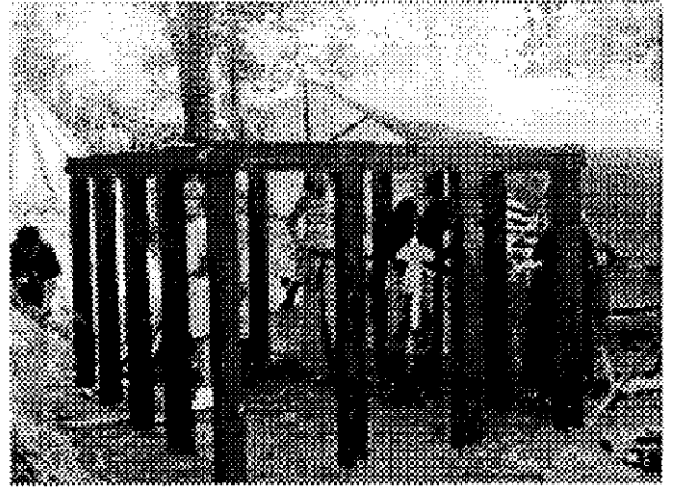
Erecting the posts and beams
